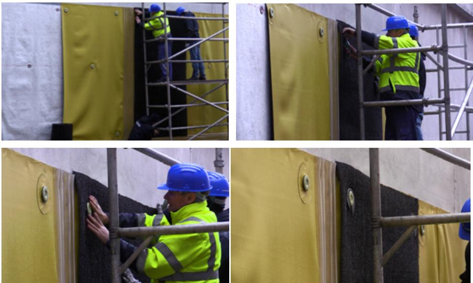
When performing vertical waterproofing from the outside (from the trench), the PETEXDREN 900 mat is laid directly on a vertical surface in stripes from top down. The PETEXDREN 900 mat is pressed by *isoweld* FI-P-6,8-PVC steel plate ([852HP Detail](#)). The rules for the position of plates are described in Paragraph 5.2.3.
